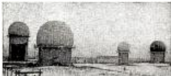
Surveillance radar towers on the DEW line. Designed for hurricane force winds and heavy ice and snow loads. These are some of more than 1000 radar towers built by Dresser-Ideco for the nation's aircraft warning system.
